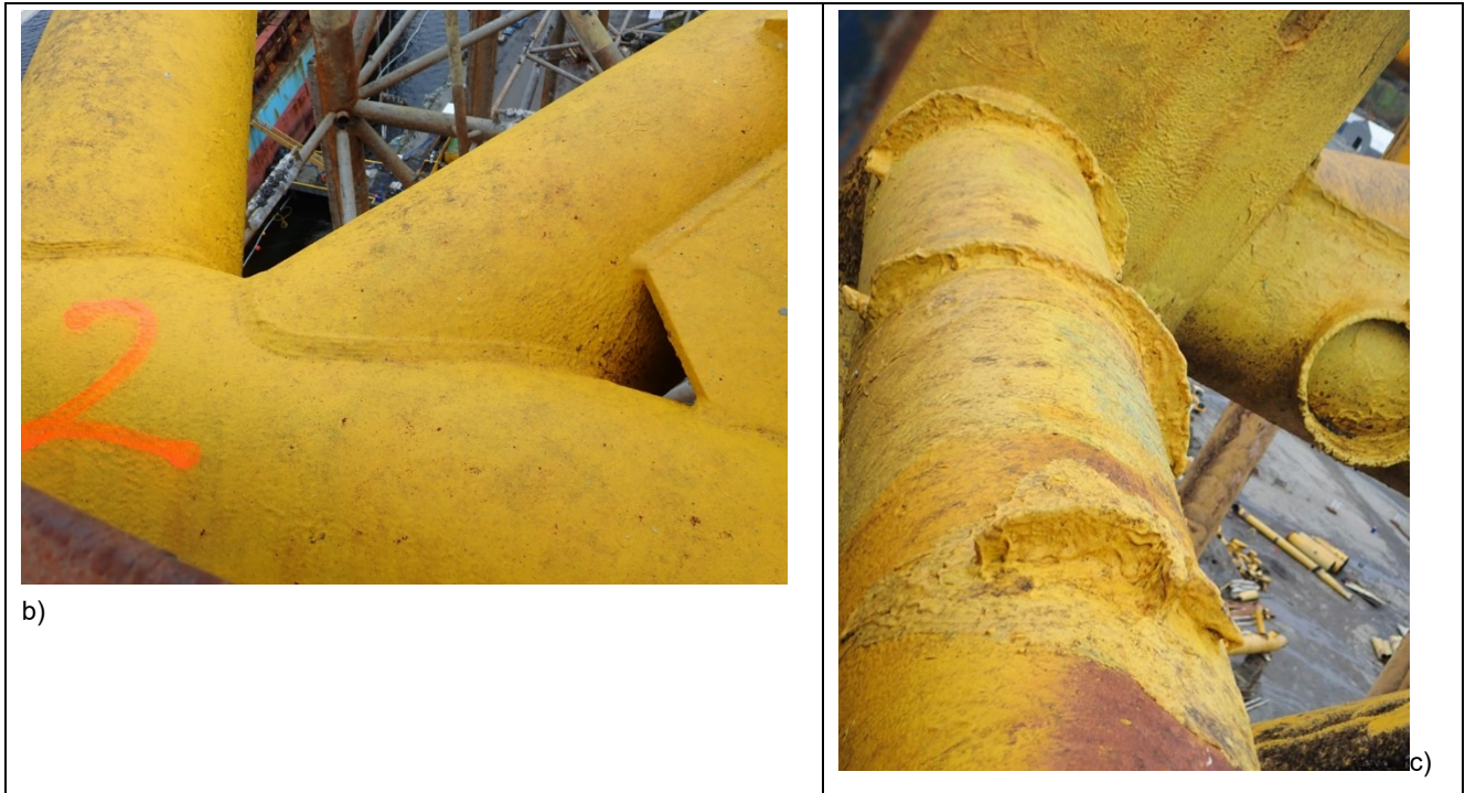
Figure 6-3 Coating appears generally good in splash zone. a) overview El. +20' (+6.1 m) from Row B. b) Close up of node at El. +20' Row 4. c) Close up of node at El. +20' Row A. Some repaired coating on steel inserts (walkway removed in 1993). Ref. /16/.
