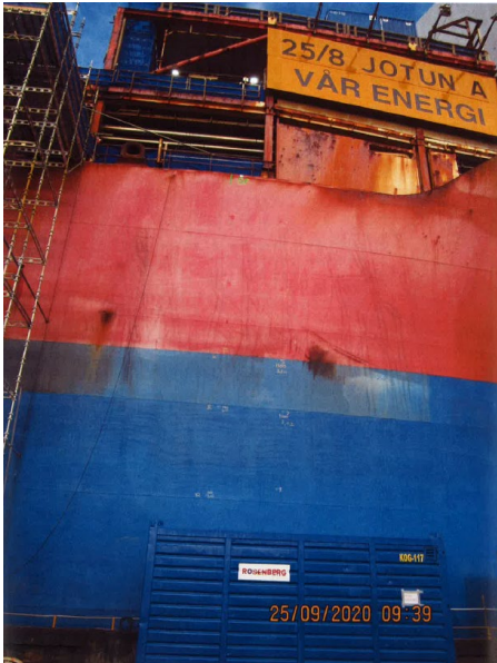
Figure 5-1 Photos of Jotun A hull starboard side, ref. /13/
